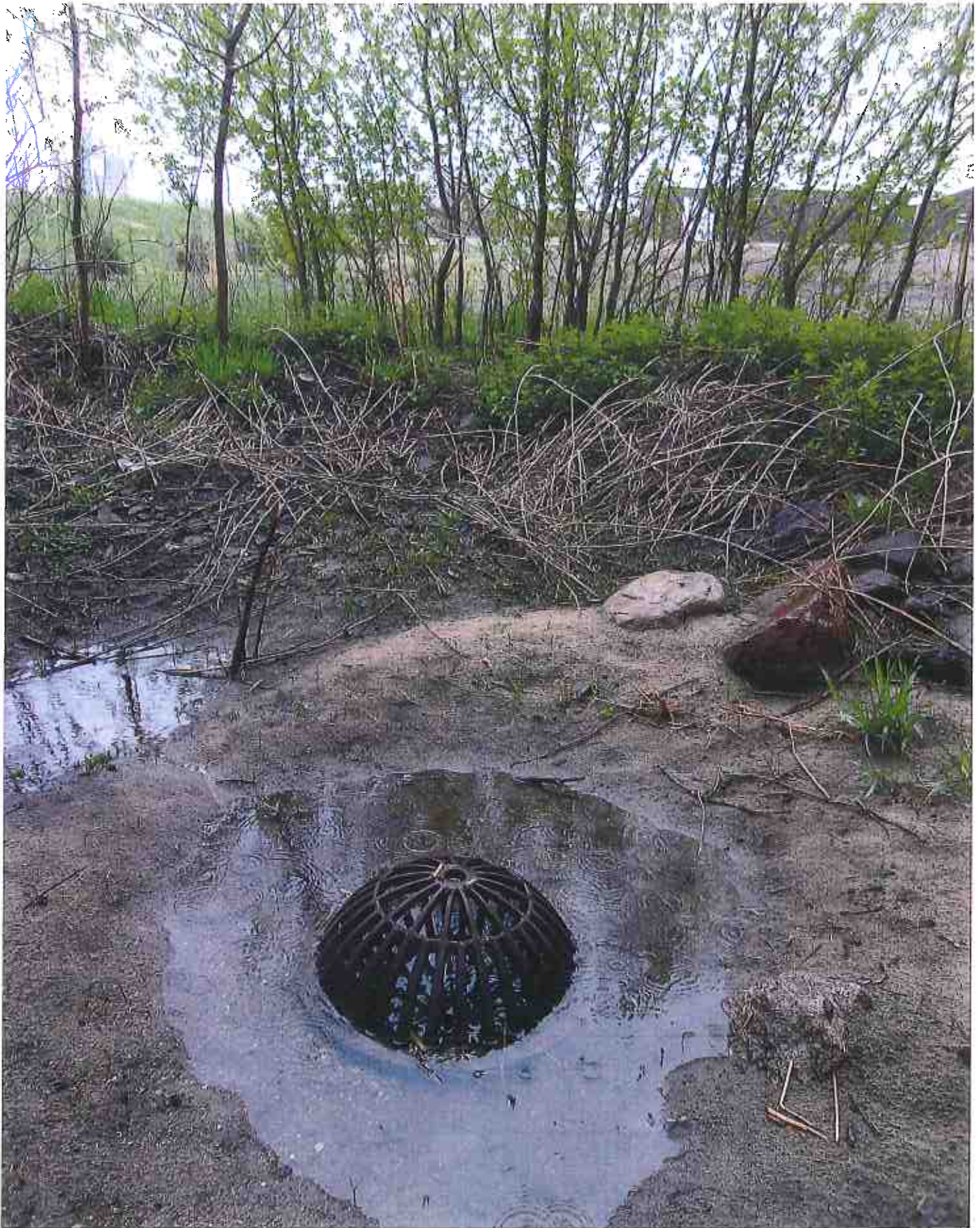
BEEHIVE OVERFLOWING @ NE COR OF GEORGETOWN ADD.
