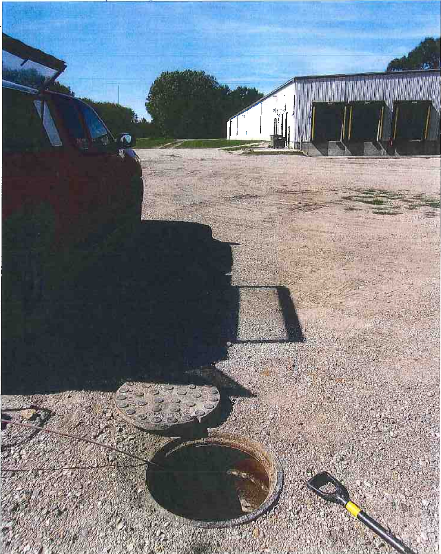
Looking W. (upstream) @ MH # 3513
