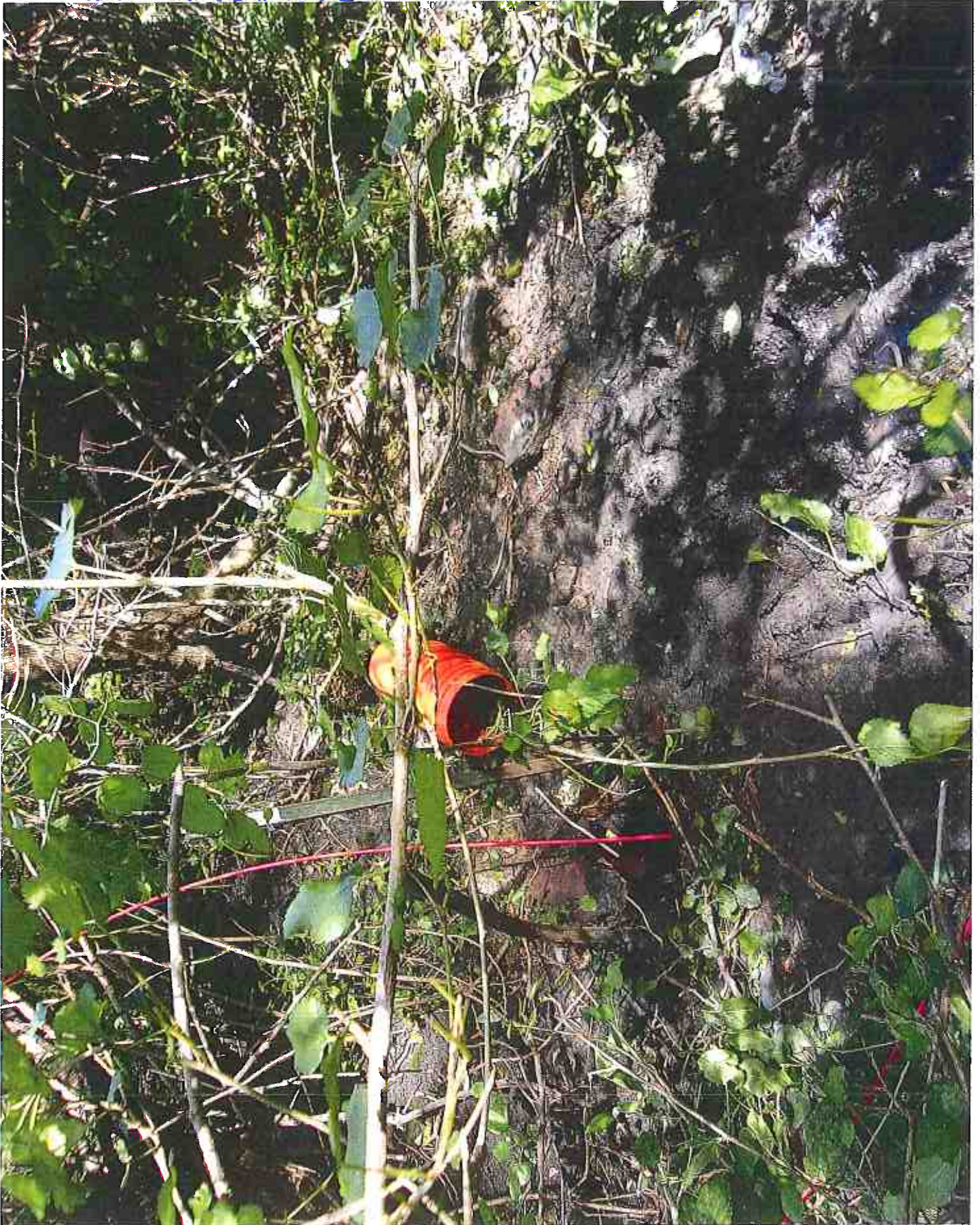
LOCKING N. (UPSTREAM) @ HICK INTAKE ON CLAY TILE #8491
