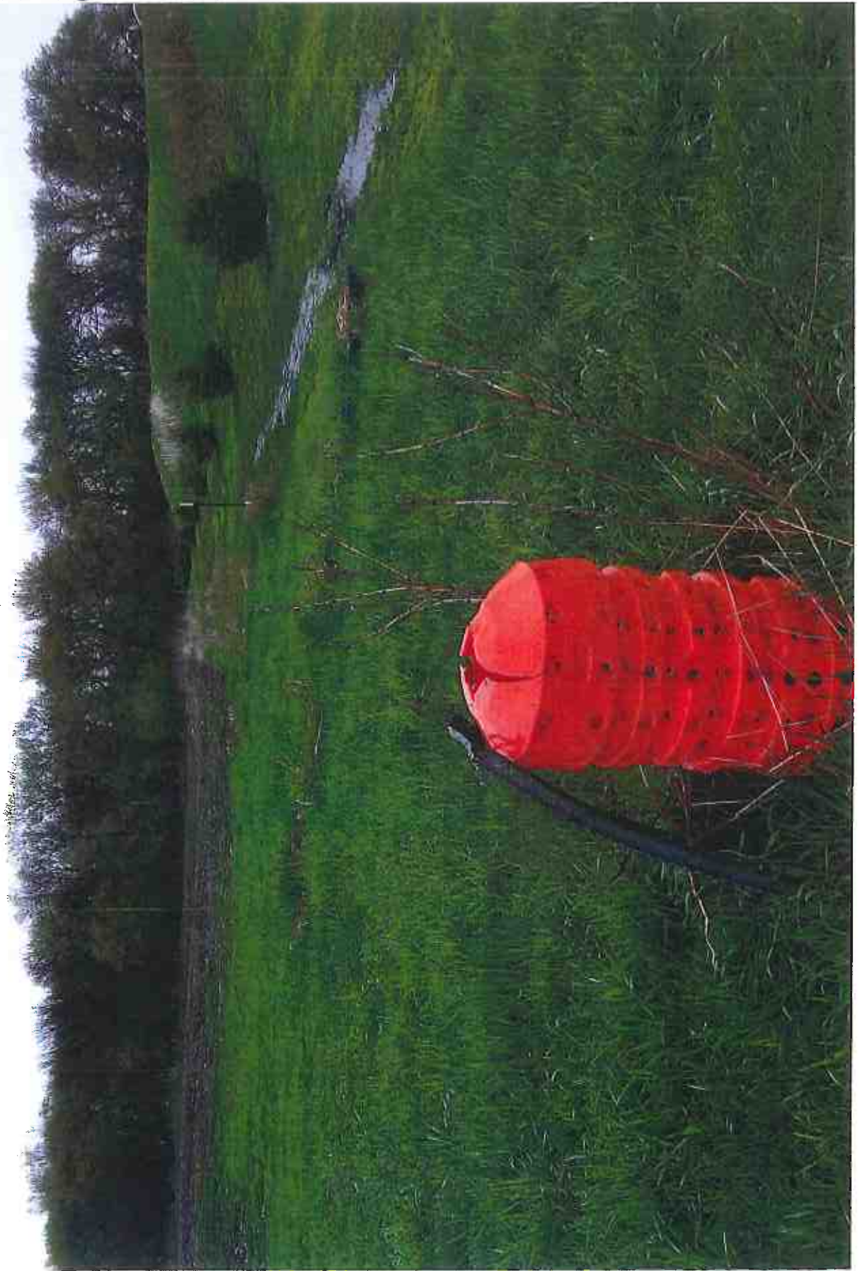
12" HICK INTAKE FULL OF WATER, SWIRLING
