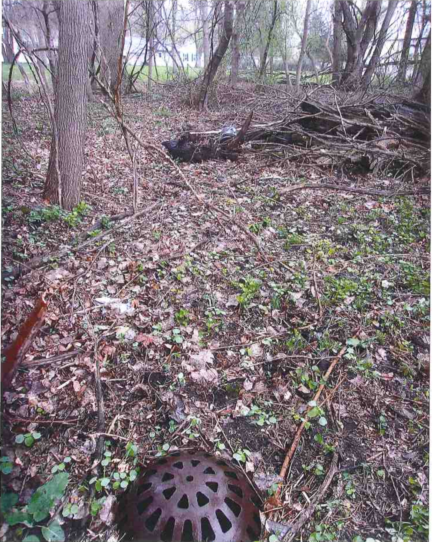
LOOKING EASTERLY FROM BEEHIVE TO OUTLET IN CITY STORM SEWER
